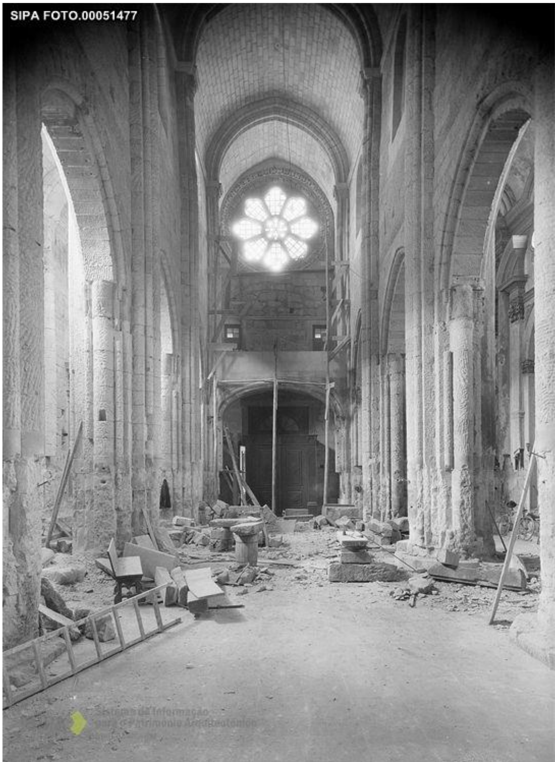
Figure 37. Central nave of the Porto Cathedral during restoration work. PCIP/SIPA FOTO.00051477, José Marques Abreu Júnior, 1933.
