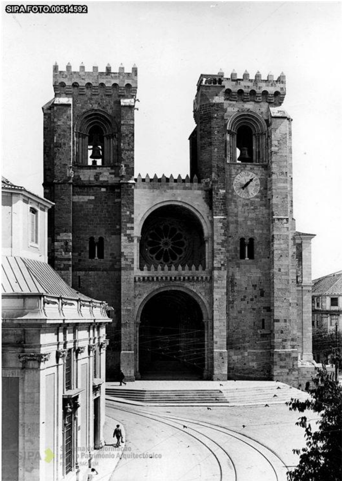
Figure 4. Main façade of the Lisbon Cathedral during restoration work under António do Couto Abreu, c.1929–1932. PCIP/ SIPA FOTO.00514592, Eduardo Portugal, undated.
