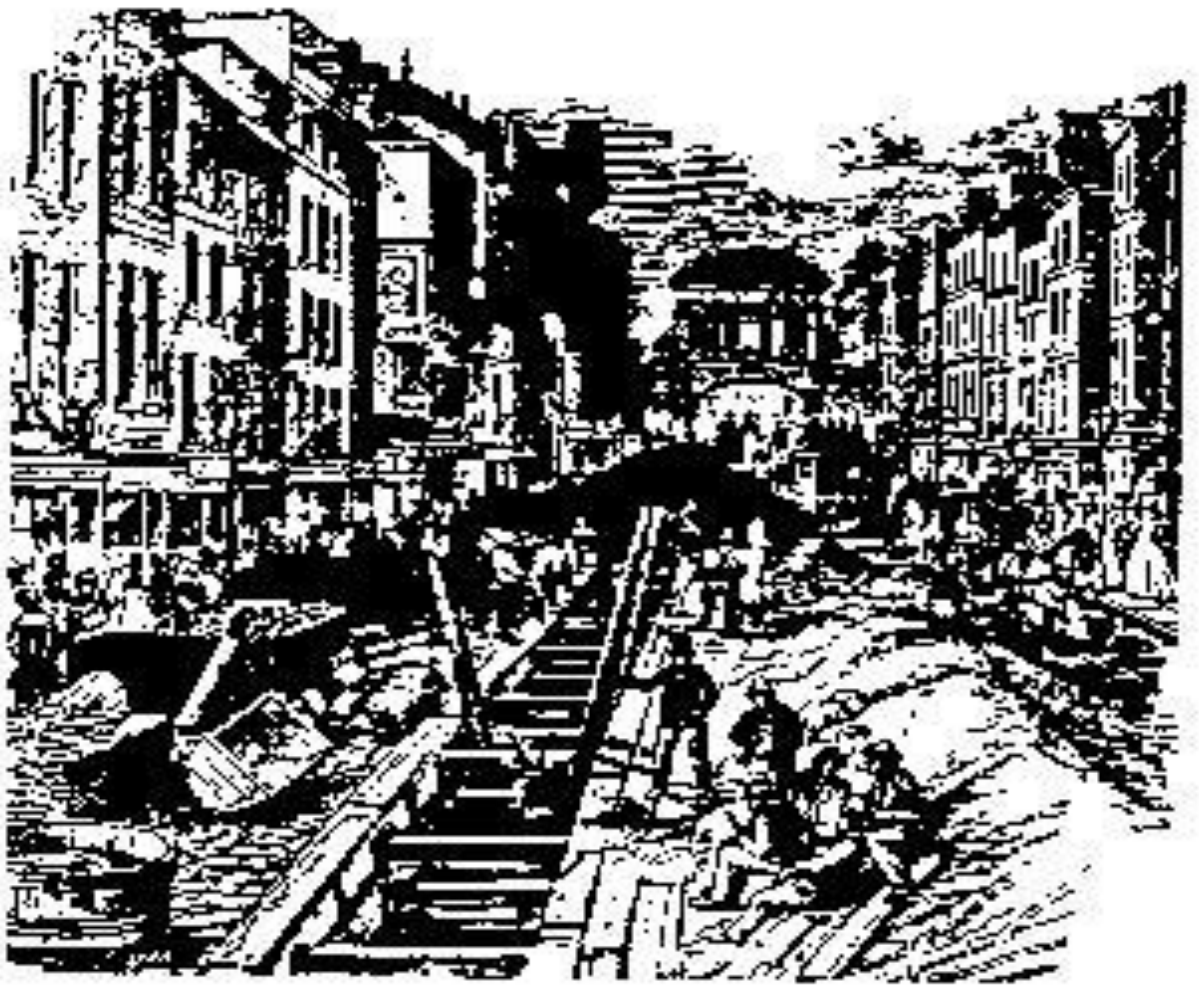
Construction of London's main sewer began in 1844
