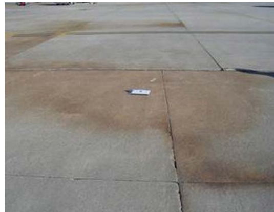
NO DEFINED LEVELS OF PUMPING
