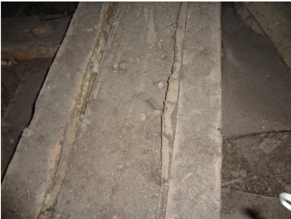
Fig. 4.22 – Tie beams entrapped by one additional timber element on each side.
