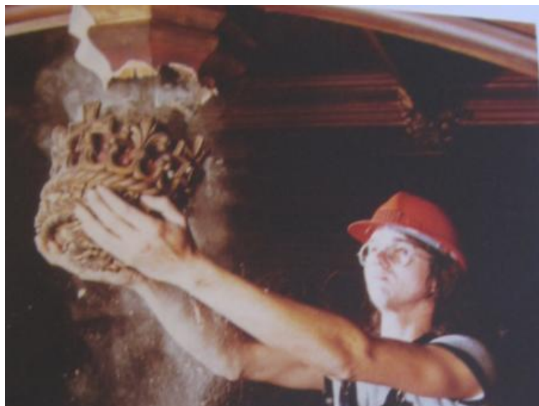
Fig. 3.4 – Heat damage – House of Lords [1].
