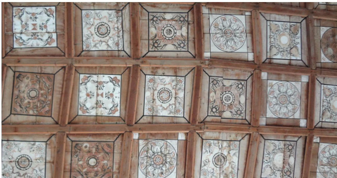
Fig. 4.6 – Painted paneled ceiling details.
