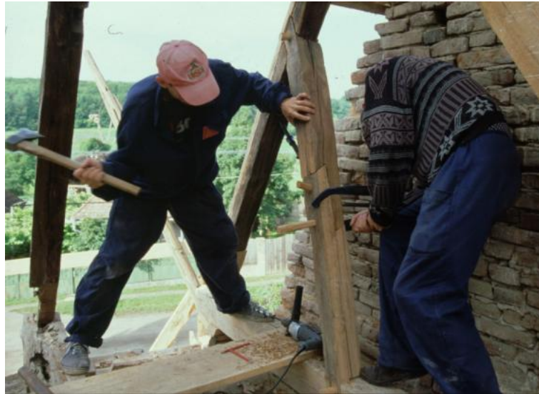
Fig. 3.27 – Timber to timber repair in situ.
