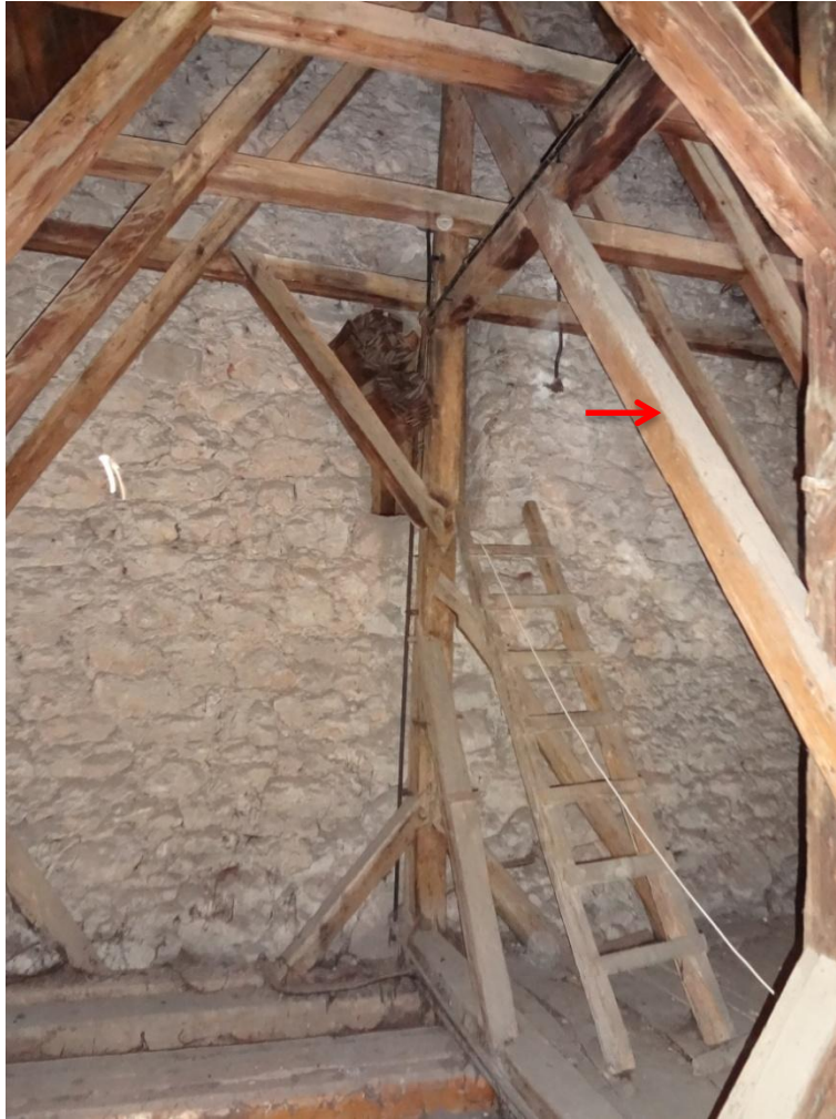
Fig. 4.19 – Replaced longitudinal passing brace.
