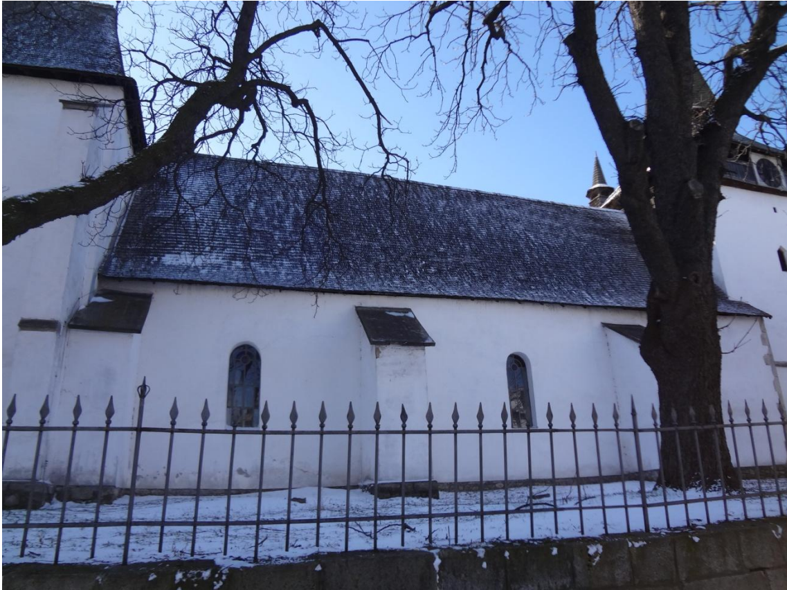
Fig.4.3 – Church nave, north side.
