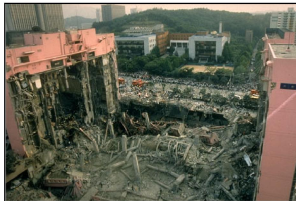
Figura 1.2: Colapso do Sampoong Department Store [38].
