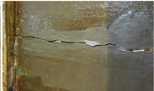
Figure I.1b: Detail of join on left side showing the wide crack in the infill used in the previous treatment and unsaturated colours from the previous reintegration.
