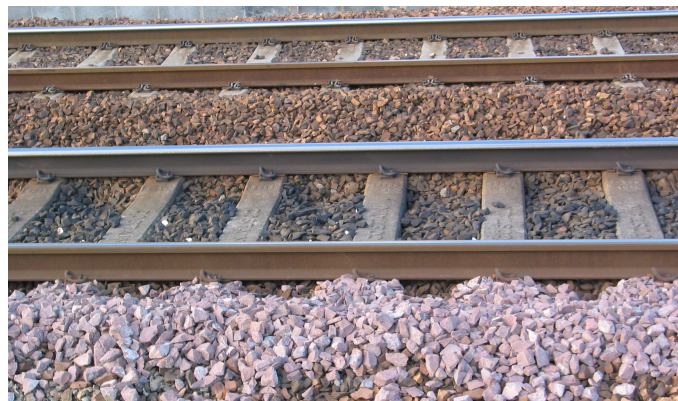
Figure 2.13: Ballast bed packed around mono-block concrete sleepers, Wikimedia Commons, 2005.
