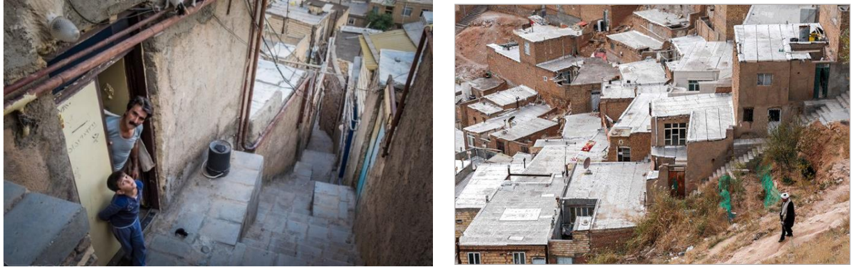
Figure 15. Ahmad Abad s in Tabriz, High Fire Risk, Limited Accessibility
