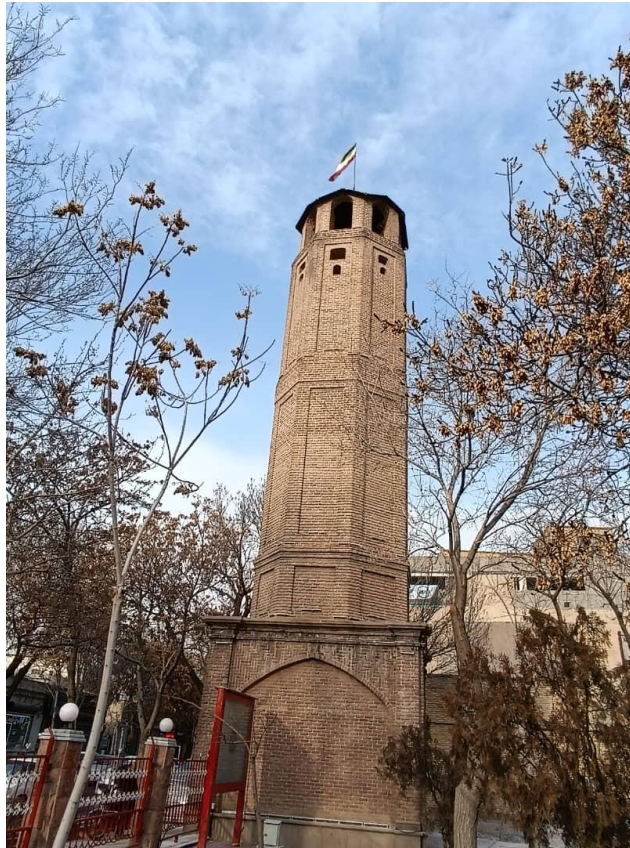
Figure 3. Fire Fighting Tower in Tabriz (Yanghyn Tower)
