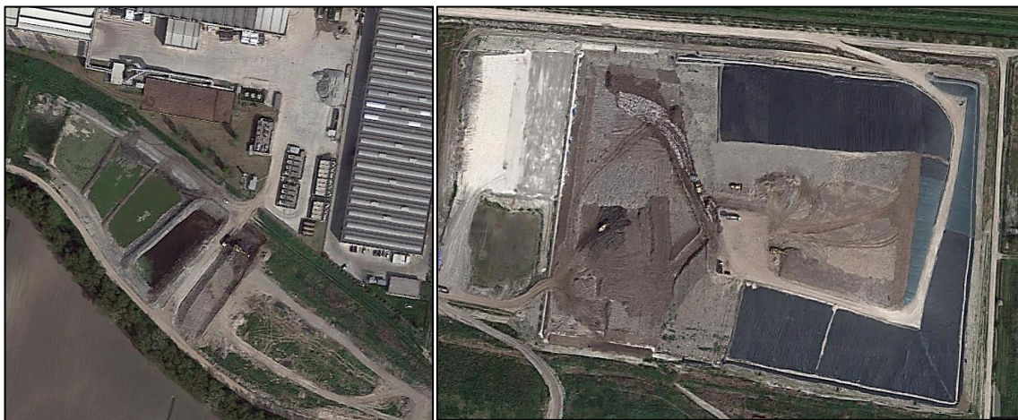
Figure 3.1 - Old sector without protective systems (on the left) and the new sector according with the legislation criterias (on the right) (Google Maps, 2017)
