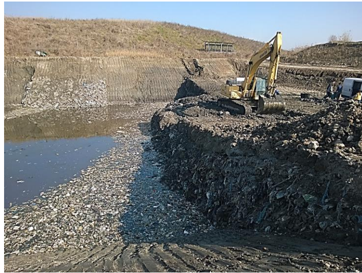
Figure 3.2 - Excavation layer for the MSW samples in study
