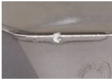
Figure 2.22: Edge chipping - Example [41]
