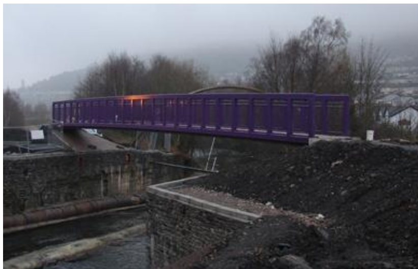
Figura 2.10 - Ponte pedonal no Riverside Park, concebida com viga Vierendeel, no Reino Unido [31].
