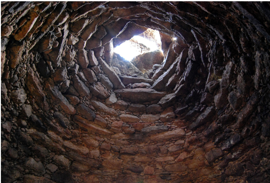
Fig. 5. Top: Alto da Cumeada's chafurdão , one of the largest examples of this form of vernacular architecture preserved in Castelo de Vide; bottom: detail of the corbelled dome, seen from below (© Fabián Cuesta-Gómez and Sara Prata).
