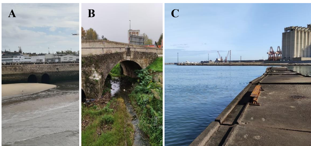
Figure 1.1. Possible examples of point and non-point source pollution in the Lisbon Metropolitan Area. (A) A sewage discharge point that leads to the Tagus River in Algés, Oeiras. (B) An open sewer pipe below the bridge arch, in Ribeira do Carenque, Amadora. (C) An industrial complex next to the Tagus River in Barreiro, Setúbal.
