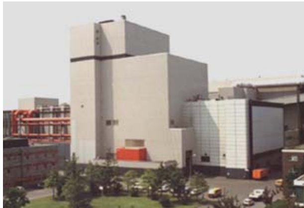
Figure 2.14 – Duisburg power plant
