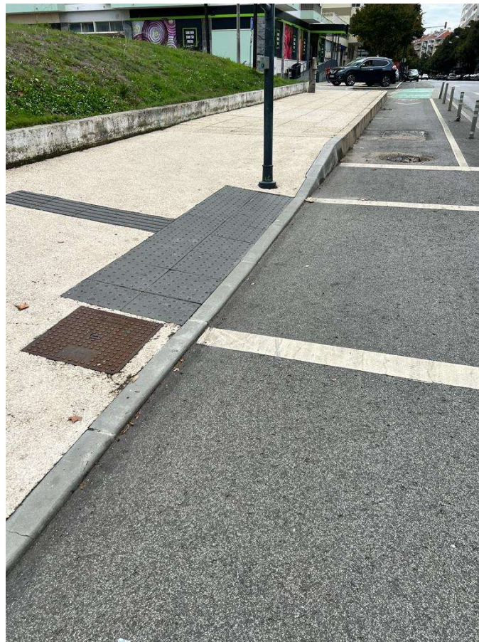
Figure 5.57 Lowered sidewalk with tactile pavement.
