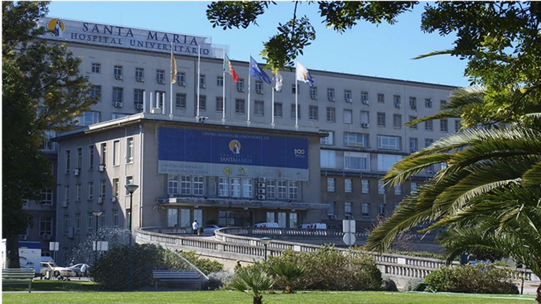
Figure 5.27 Santa Maria hospital.
