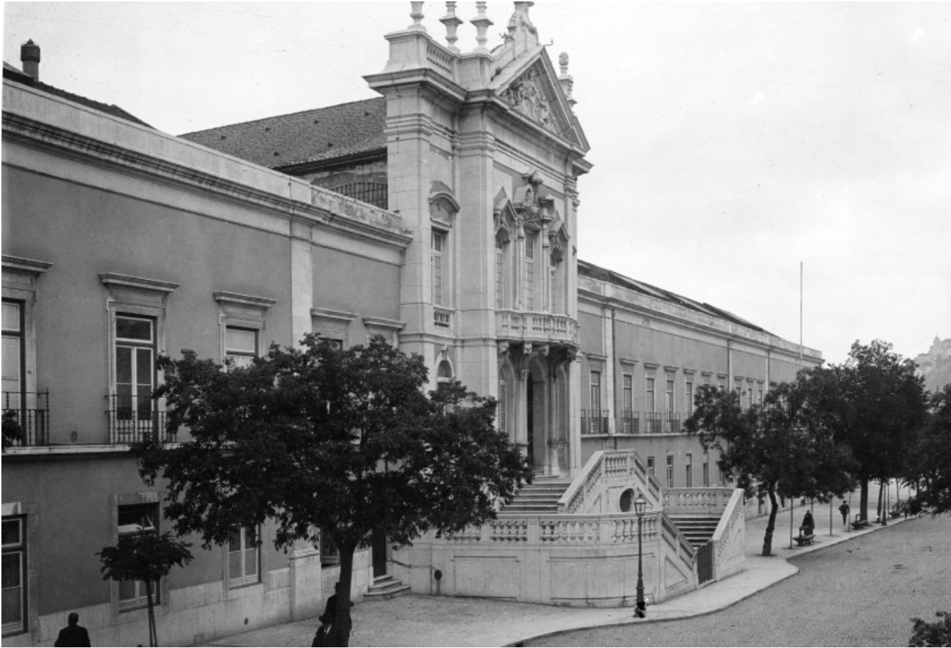
■ Main façade of Bemposta Palace, home to the Army School from the late 1850s. [B&w photograph by J. Benoiel (19--). AML – NF]
