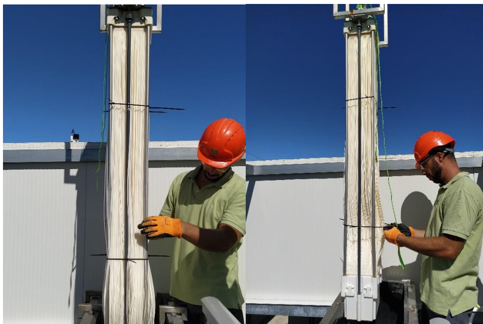
Figure 4.6 – Membrane removal.
