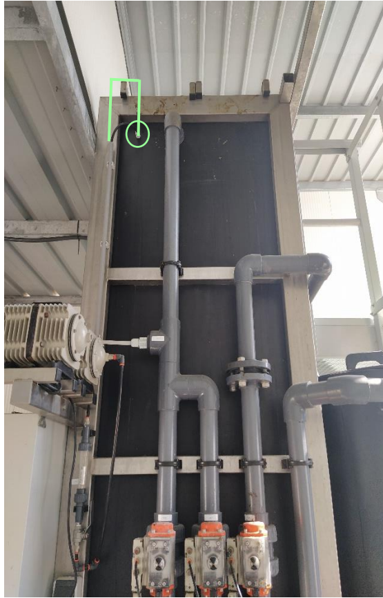
Figure 4.1 – Blower connection to the concentrator tank.
