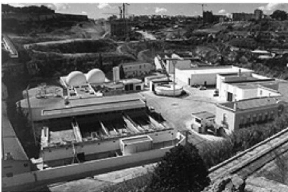
Figure 2.1: Full view of Chelas Sewage Treatment Plant.
