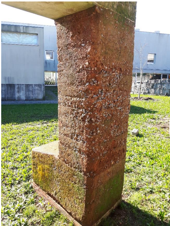
East view (corresponding to the cut view in the drawings) before intervention
