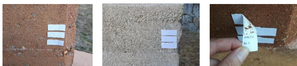
Figure 6.11: Scotch tape test on both columns of unstabilized and stabilized earthen material.
