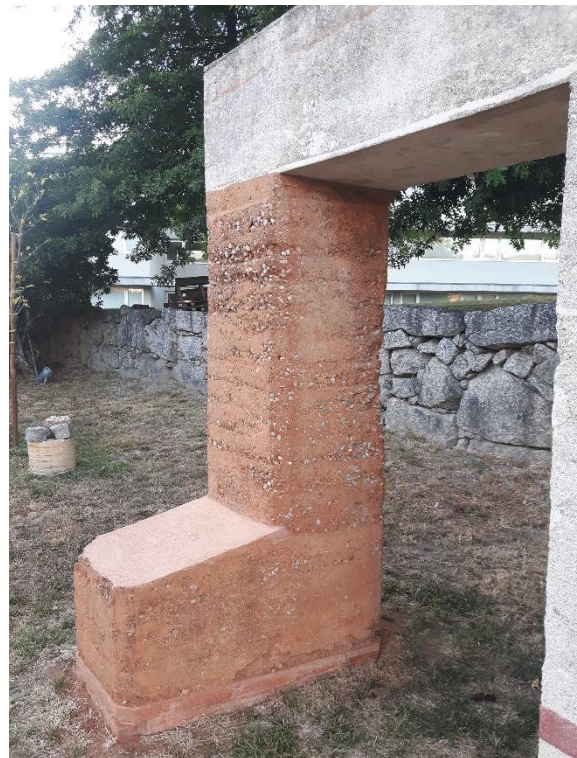
East view (corresponding to the cut view in the drawings) after intervention
