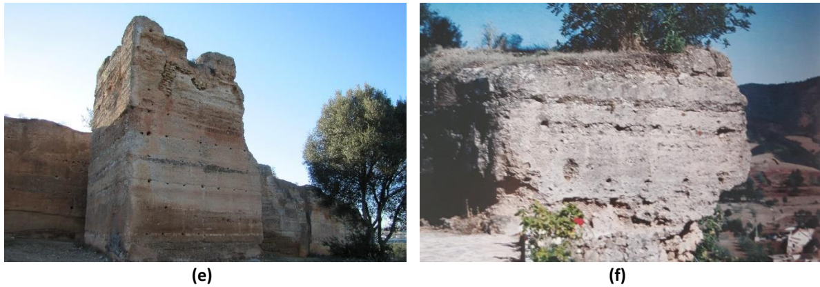
Figure 2.15: Examples of castles built with military rammed earth in Portugal. (a) Alcácer do Sal ( credits: (Torres and Macias 1998) ); (b) Juromenha ( credits: (Torres and Macias 1998) ); (c) Moura ( credits: (Torres and Macias 1998) ); (d) Silves ( credits: (Torres and Macias 1998) ); (e) Paderne ( credits: Daniel Oliveira ); (f) Salir ( credits: (Torres and Macias 1998) ).
