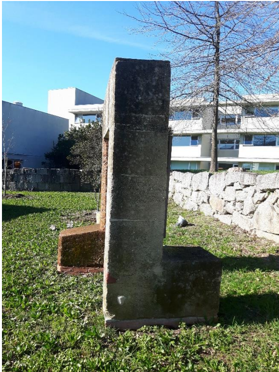
East view before intervention
