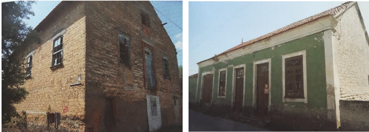
Figure 2.17: Examples of adobe construction in Aveiro (credits: (Fernandes and Tavares 2016)).
