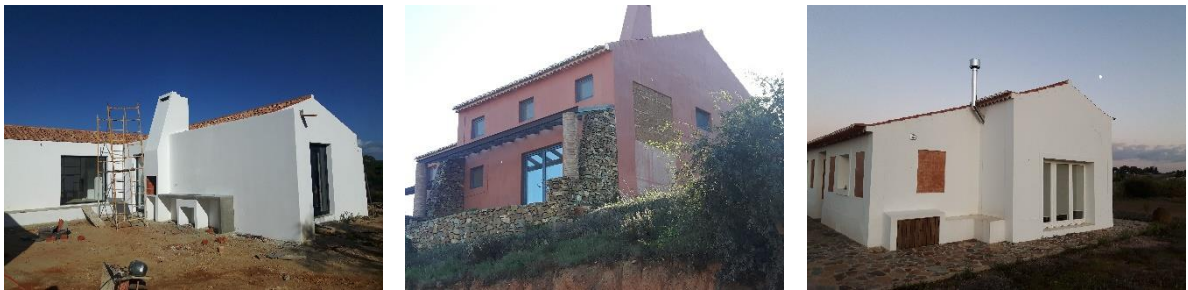
Figure 2.16: Three examples of new construction (2019) in Alentejo made with traditional rammed earth technique.
