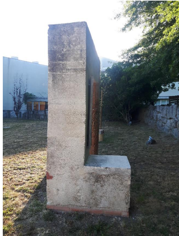
East view after intervention
