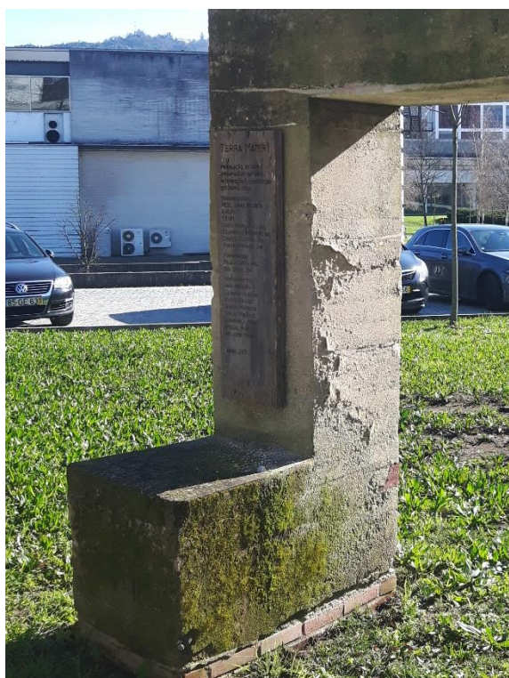
West view (corresponding to the cut view in the drawings) before intervention
