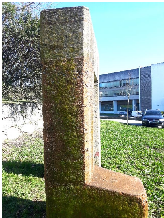
West view before intervention
