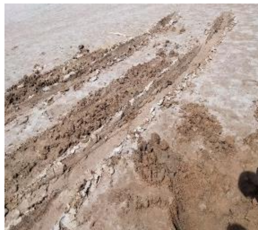
Figure 10. Damage caused on sebkha surface by wheels.
