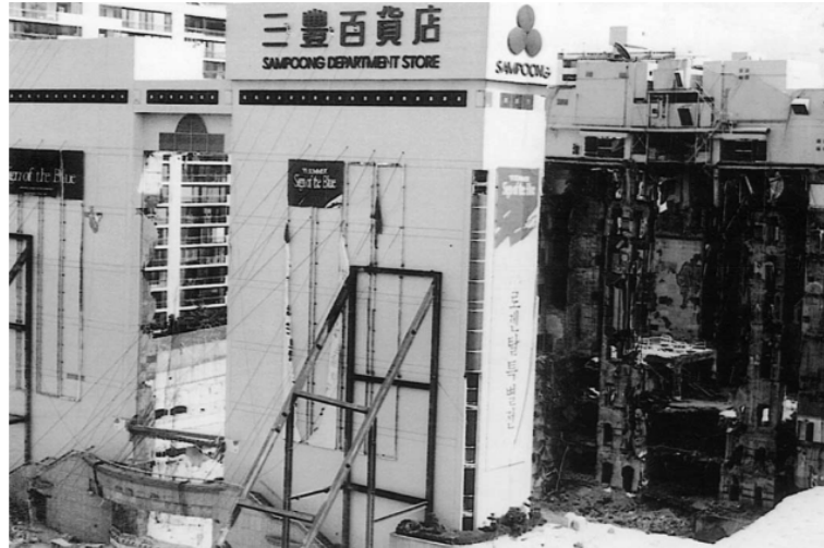
Figura 2.3 – Destroços do Sampoong Department store, Gardner et al (2002).
