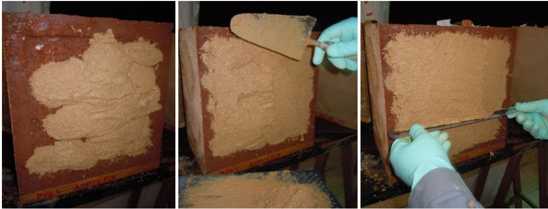
Figure 2: Application of the mortar MRE_AL15 on a standard superficial defect of the PD rammed earth
