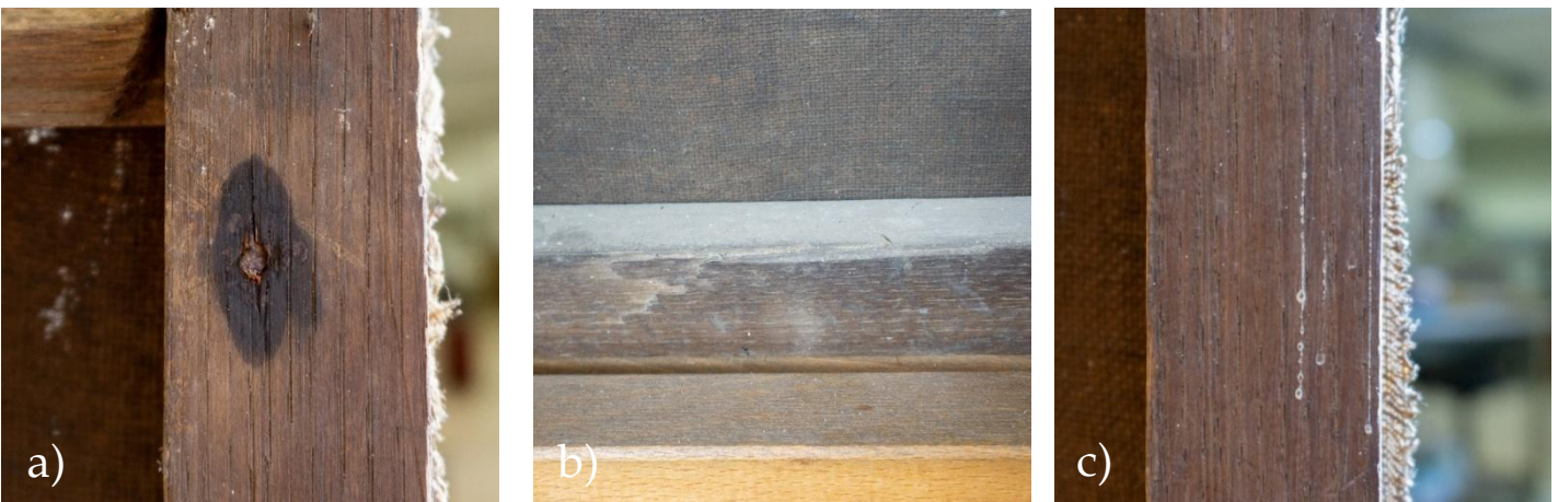
Figure D.4: a) Stain surrounding a rusted tack; b) Deposited dirt on the lower strainer member; c) White stain, possibly white paint on the right side of the strainer.
