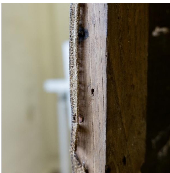
Figure 2.8: Tacks that do not provide tension to the canvas.
