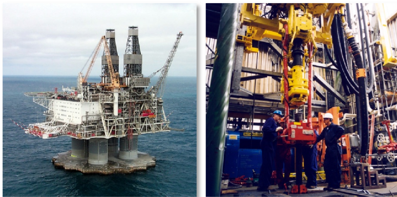
Figure 1.1: The Hibernia oil platform rig, one of the world's largest (Hibernia, 2009).
