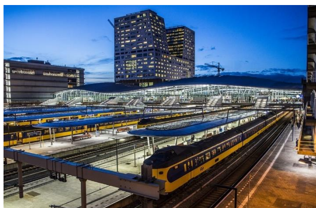
Figura 10 Utrecht Central Station
