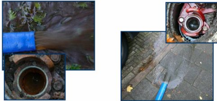
Fig. 5-6 Brown water coming out of the cast-iron pipes (on the left) and clear water from PVC (on the right)
