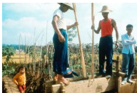
China - Ramming a wall Photo unknown
