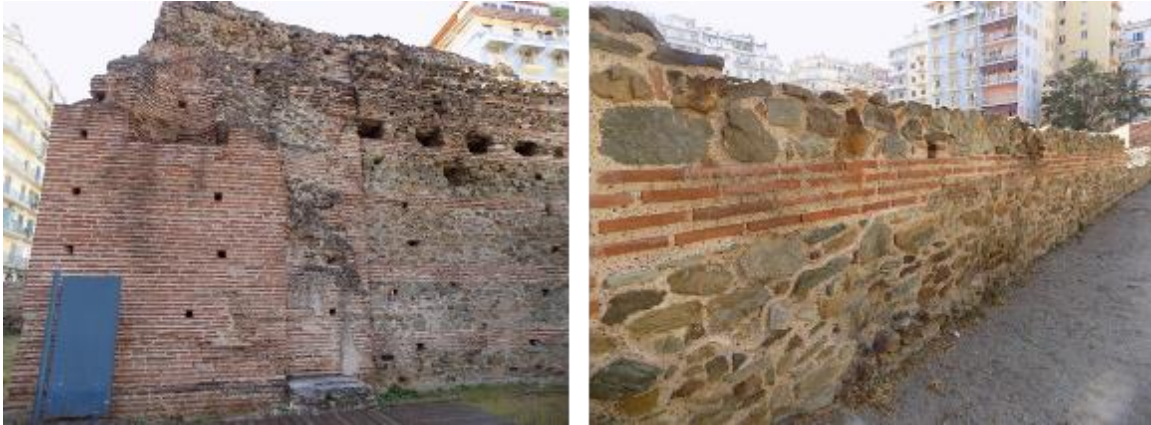
Figure 13. Repaired masonries of Galerius Palace, as they are now.
