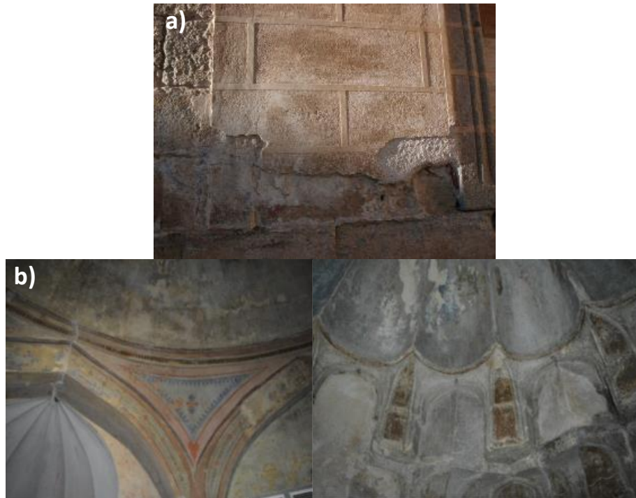
Figure 3. a) Durability of air lime render imitating stone over stone masonry in Évora Cathedral, in Portugal (17th century); b) Interior of Pasa Hamam, Thessaloniki (1530 AD), with well-preserved air lime renders ( \text{CaO} \geq 55\% ) although soluble salt content was high \geq 1\% .
