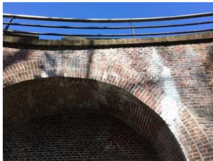
Figure 33. Arch section in the masonry of the motte castle of Leiden, after reconstruction of the section.
