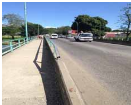
Figure 8. Metaniko Bridge 2-Lane exiting to Single Lane
