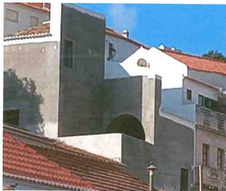
Figure 3 New dwellings in Aljezur
