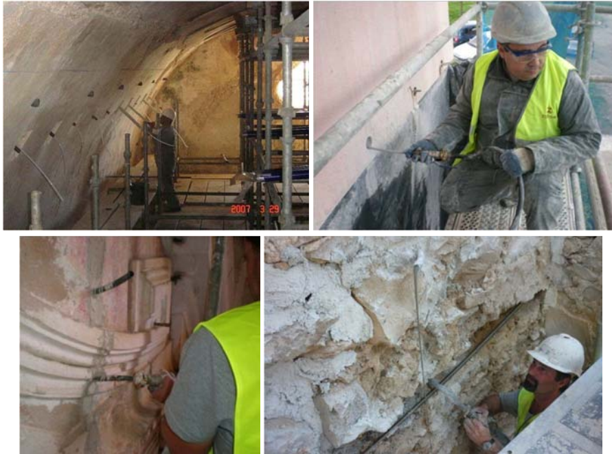
Fig. 3.5 – Masonry structures strengthened by grout injection (photos from ZIRCOM)
