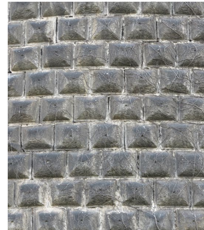
FIG. 2 Bologna medieval tower Garisenda basement, XII century. Foto by: Oxana Smagol (2014).
