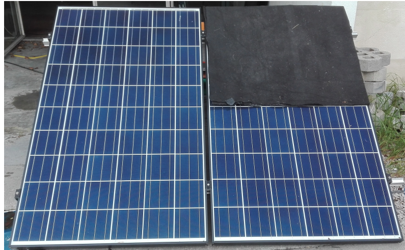
Figure 4.19: Layout of experiment 6 - Installation with an opaque fabric casting soft shade on half of the surface of a module.
