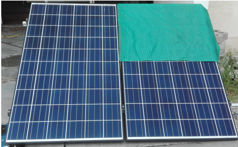
Figure 4.17: Layout of experiment 5 - Installation with a translucent fabric casting soft shade on half of the surface of one module.
