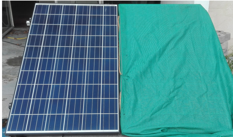
Figure 4.15: Layout of experiment 4 - Photovoltaic installation with a translucent fabric casting soft shade on totality of one module surface.
