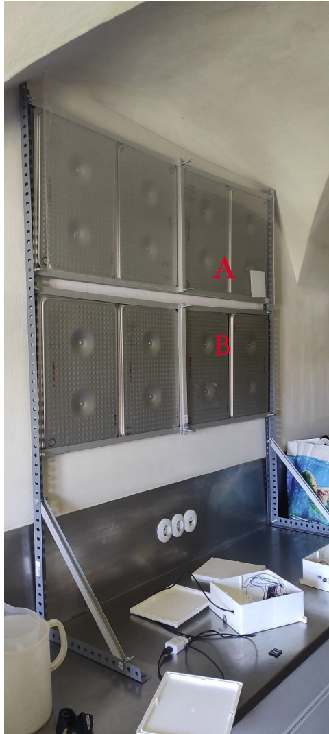
Figure 3.11: Positions of the three sensors in the structure.
