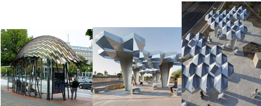
Figura 4.8 Exemplos de estruturas de altura variável. Fonte: a) Autor: Maria Kutay; b) Autor: Denis Mignoli; c) https://archinect.com/firms/project/33961/shadow-play/149996129?utm_content=buffer6075&utm_medium=social&utm_source=pinterest.com&utm_campaign=buffer#&qid=1&pid=1 .
