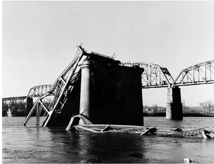
Figura 2.1: Colapso da Silver Bridge, 1967 (West Virginia Division of Culture and History, n.d)
