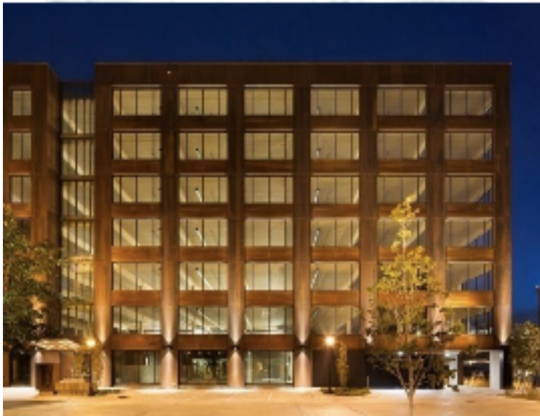
Figura 3.5: Edifício “T3 – Timber, Technology and Transit”, USA [17]
