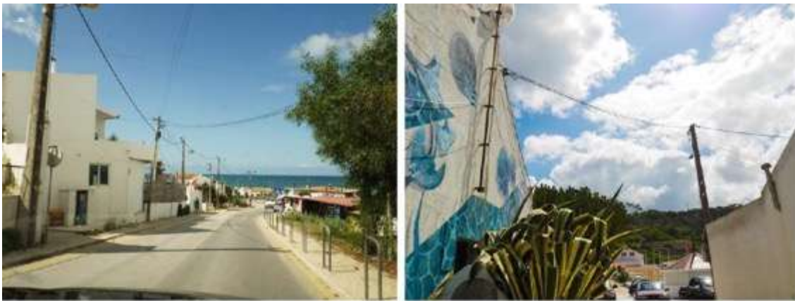
Figure 34& Figure 35- Existing conditions for Electrical Infrastructure. July 2023-Fonte da Telha, Source: Thesis Author
