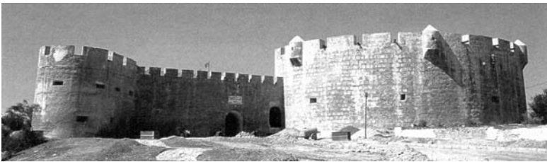
23 Semi-circular bastion of the citadel of Safim ( Borj ed Dar ), Lourenço Argueiro (1540), photo by Jorge Correia.
