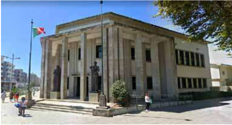
fig. I.AG 16 Raúl Rodrigues Lima (1909-1980) Palácio da Justiça da Póvoa de Varzim, 1965 Vista exterior https://www.google.com/maps/@41.3830444,-8.7599004,3a,75y,265.76h,93t/data=!3m6!1e1!3m4!1s424yE3Cs1ra2e-R1pK4mRA!2e0!7i16384!8i8192
