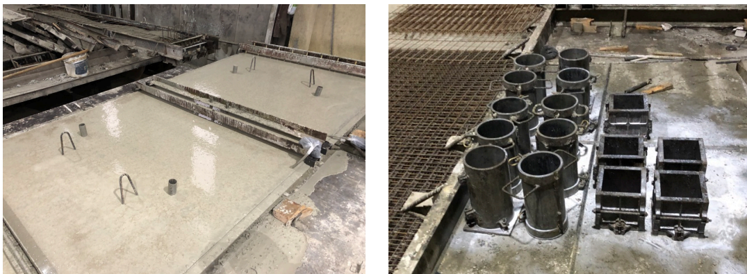
Figure 33 - Casting of the slabs, cubes and cylinders
