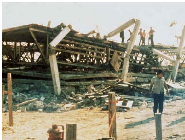
Figure 2 - Collapse of Harbor Cay Condominium in 1981 (Erdogan, 2010)
