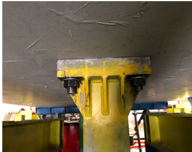
Figure 40 - Fixed column below the slab
