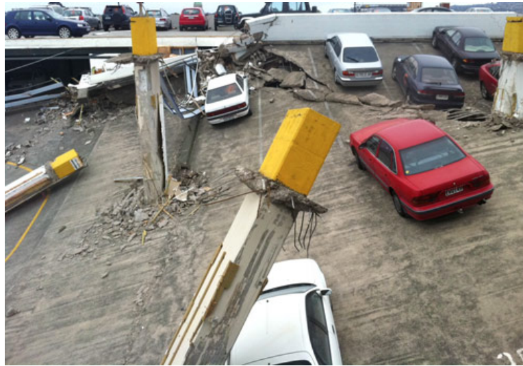
Figure 3 - Collapse of a building in New Zealand in 2011 (Swanson, 2011)
