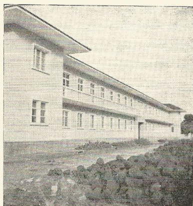
Novo pavilhão do Hospital Central de Bissau
