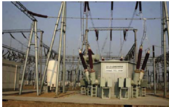
(b) InnoPower saturable-core SFCL
