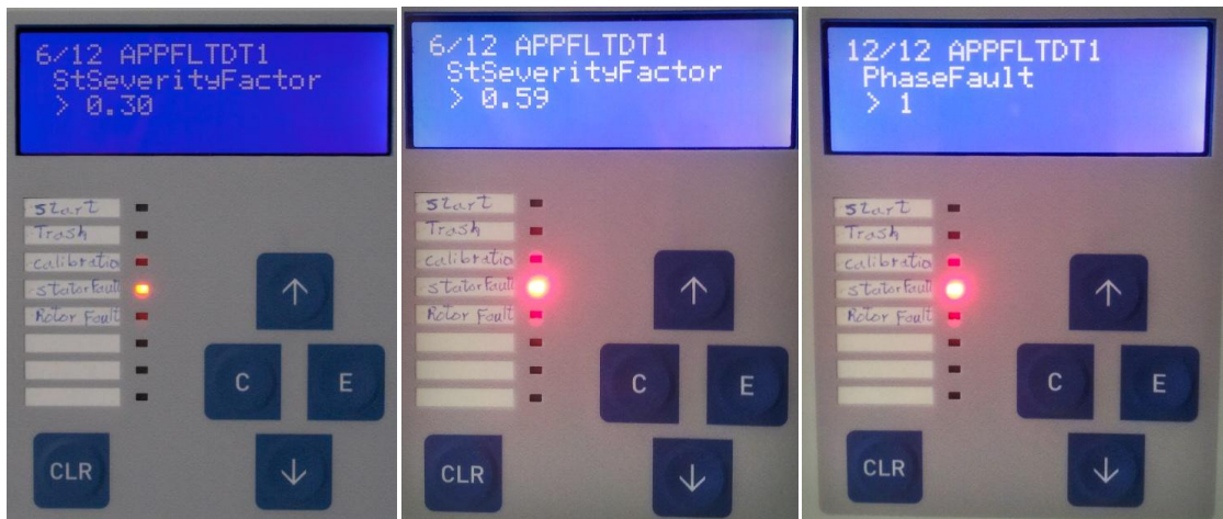
Figure 6.32 – HMI of the TPU with the indication of a stator fault in the phase 1 (A)
