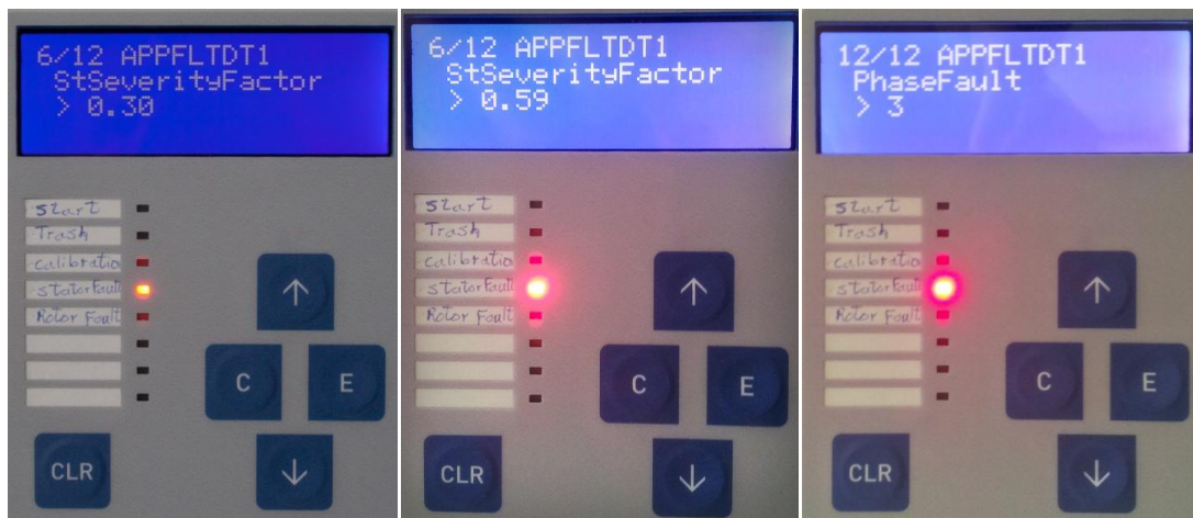
Figure 6.38 – HMI of the TPU with the indication of a stator fault in the phase 3 (C)
