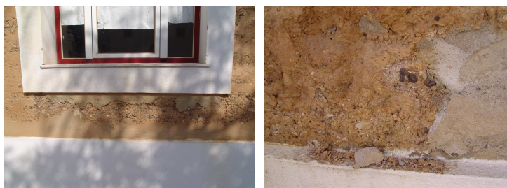
Figure 3. Rammed earth market house in S. Luís, Odemira. Left, repair with hard cement; and right, agents of degradation namely insects underneath the repair.
