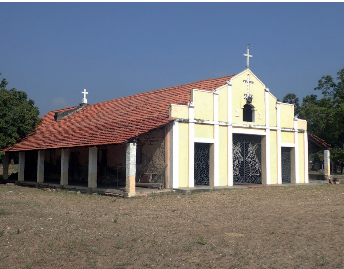
Image 46 – Exterior of the Church of St. Bartholomew, in Olaitthoduvai (source: Joaquim Rodrigues dos Santos)
