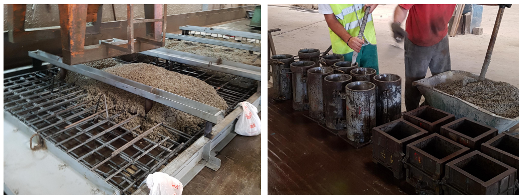
(a) Casting of the specimen
