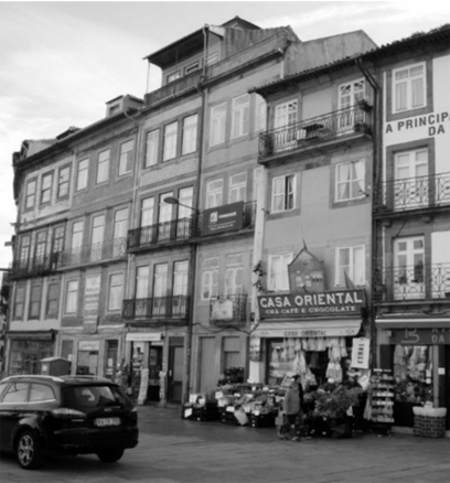
Fig. 4 - Façade in downtown Porto. Credit: Author, 2014
