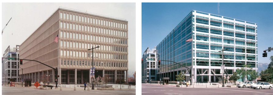
Figure 2.32: Wallace F. Bennet Federal Building, USA: (left) Before BRB seismic retrofitting, (right) after BRB seismic retrofitting
