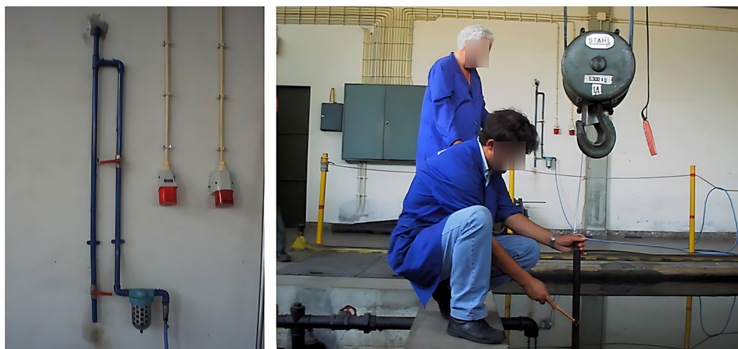
Fig. 5 The water inlet filter ( left ) and the crane used to transport cargo along the tank ( right ).
